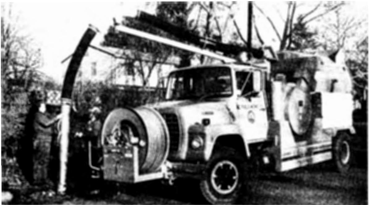
*A sewer jet cleaning truck was delivered to the DPW in November 1986. The dual-purpose vehicle is used to clean sanitary sewers and storm drains (front end) and to clean catch basins and collect leaves on unimproved streets (back end).*
